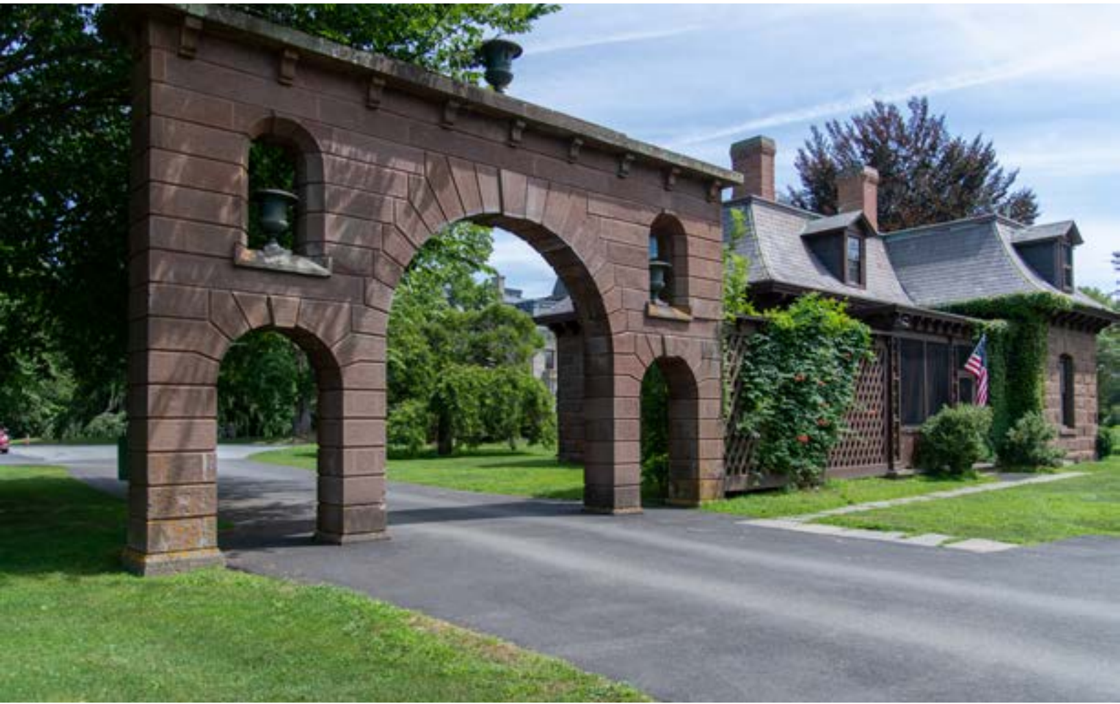
Chateau gate house
